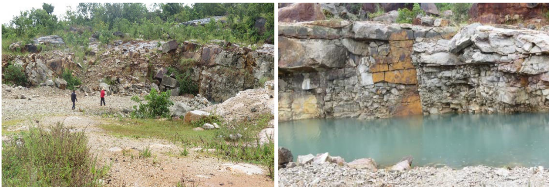
Figure 7-5 Overlying Early Coarse-grained Granite (left) and Underlying Late Fine-grained Granite (right) with a Gently Northward-dipping Contact in a Quarry
